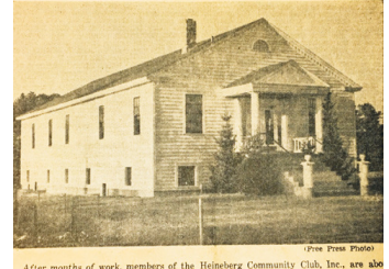
After months of work, members of the Heineberg Community Club, Inc., are about to complete their clubhouse shown above. Although not entirely finished, the building is ready for occupancy.
